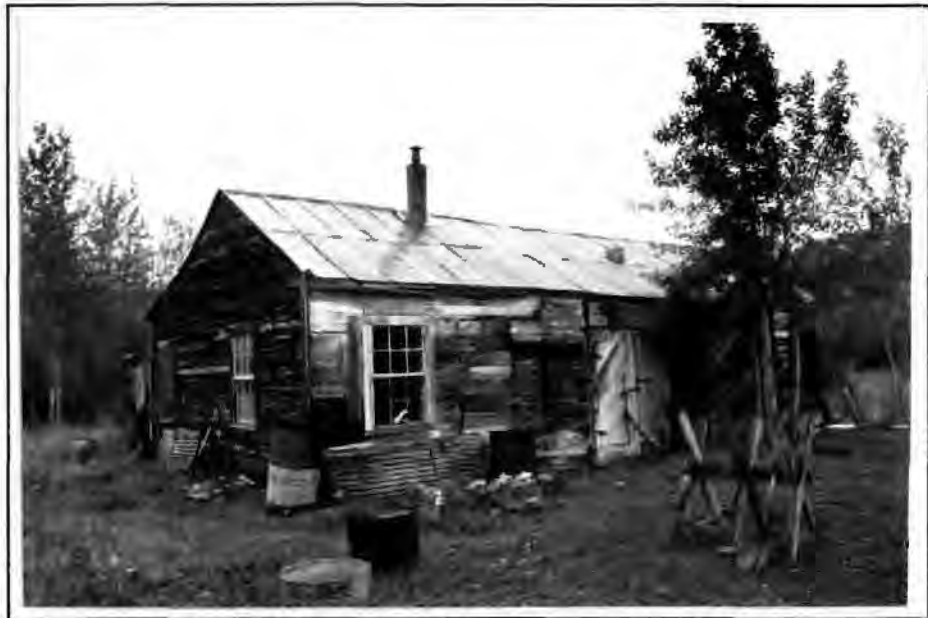
Figure 129. The ARC Repair Shop, 1993. The view is looking northwest.
